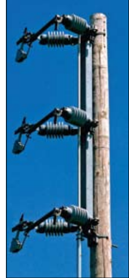
Phase-over-Phase Mounting
